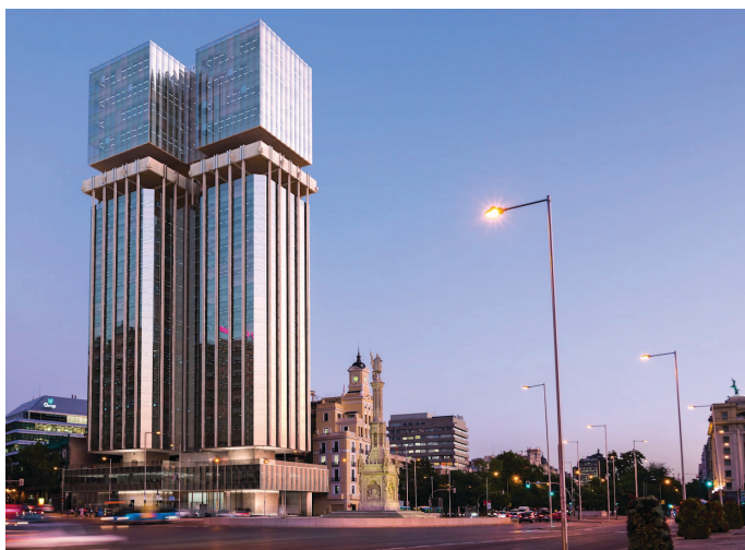
Comprehensive reform project for the Colón Towers (Madrid), which continues with the participation of Hill.
